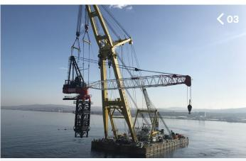
NOVEMBER 2019: Using a 2,200-tonne capacity Taklift 4 floating heavy barge crane, the cranes – each weighing 600 tonnes – were lifted from the quayside and transported to the worksites a kilometre off-shore on the Çanakkale Strait. It was the first of two world-first engineering feats on the project.
