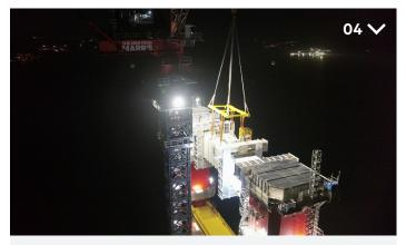
JUNE 2020: After climbing the cranes to their final height of 328 metres, the next major milestone was the installation of the upper cross beam (UCB). With the M2480D positioned 328 metres above the water, it took approximately 30 minutes (and a lot of planning) to lift the 155-tonne section into position – creating a new world record for the heaviest lift (155 tonnes) at height (318 metres).
