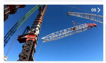
JULY - AUGUST 2020: After successfully completing the construction of the bridge towers, the M2480D HLLs were climbed down the completed bridge towers and safely recovered.
