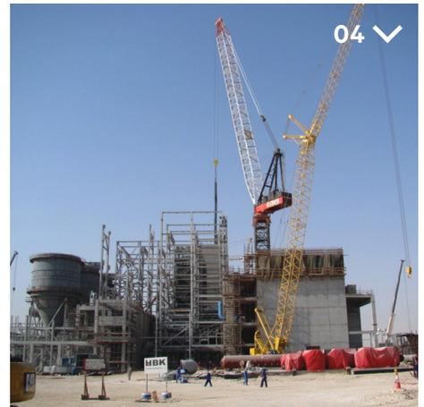
**MAY 2008:** 12-months later we had built the crane in Australia and shipped it to Doha. With the M2480D doing all the heavy lifting from the perimeter of the site, there was no longer any need to shut down parts of the construction site. Productivity increased by 30-50%.
