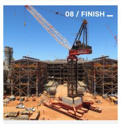
**NOVEMBER 2013.** 18 months later the SMPT trailer solution we used to load the M2480D was employed at the LNG Plant to move tower cranes around the construction site.
