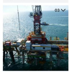
Marr was contracted by McDonnell Dowell to develop a complex cranage system for building a cyclone-proof structure and ongoing support infrastructure in open waters 2km out to sea.
