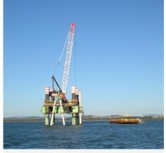
Using Sante Fe jack-up barges (JUB) as movable work platforms, we set up the first M2480D crane on the JUB and towed it from Mackay Harbour to the construction site to build the first of the M2480D travelling wharf cranes. The first M2480D wharf crane was subsequently used to install the second and third M2480D travelling wharf cranes.
