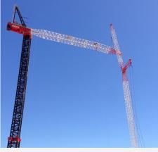
Capacity of the Liebherr LR 1280 erection crane meant that the boom had to be lifted in two pieces. The first half was hung off the erection pendants with the second half lifted into position and held while the crane luffing system was reeved.
