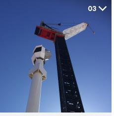
We engineered a solution that allowed the crane to free-stand without the need for counter-weight ballast at the base of the crane. This solution saved the client the expense of having to transport any counter-weight ballast to and from site.
