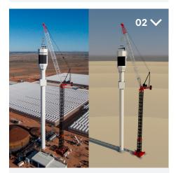
We used 3D computer modelling to check our solution and assist with the development of the install methodology and critical lift plans. (Image of 3D modelling against final lift).
