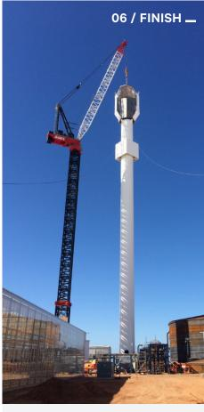
For the final lift to install the drum on the top of the tower, John Holland and our rigging team developed a system of taglines attached to winches to prevent the load from spinning as it was lifted 100-metres off the ground.
