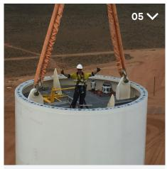
Part of our crane install rigging team stayed onsite to operate the crane, complete all the critical lifts and the rigging works associated with installation of the solar tower.
