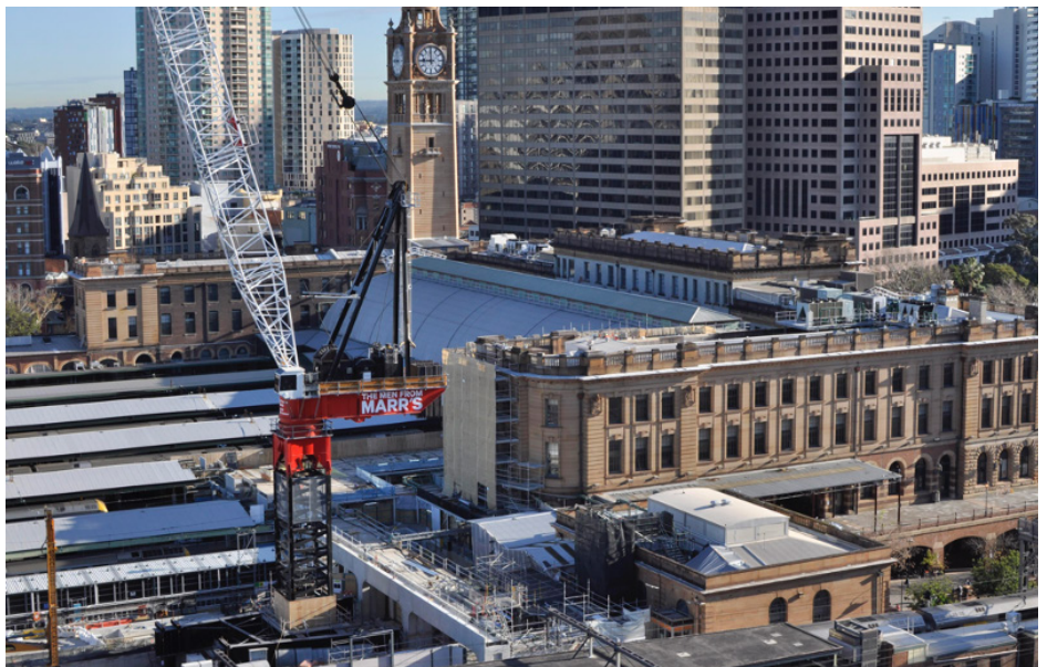
Marr's M1680D HLL was installed at Central Station to complete heavy lift and general construction requirements on above and below ground works associated with the redevelopment of Australia's busiest railway station.
