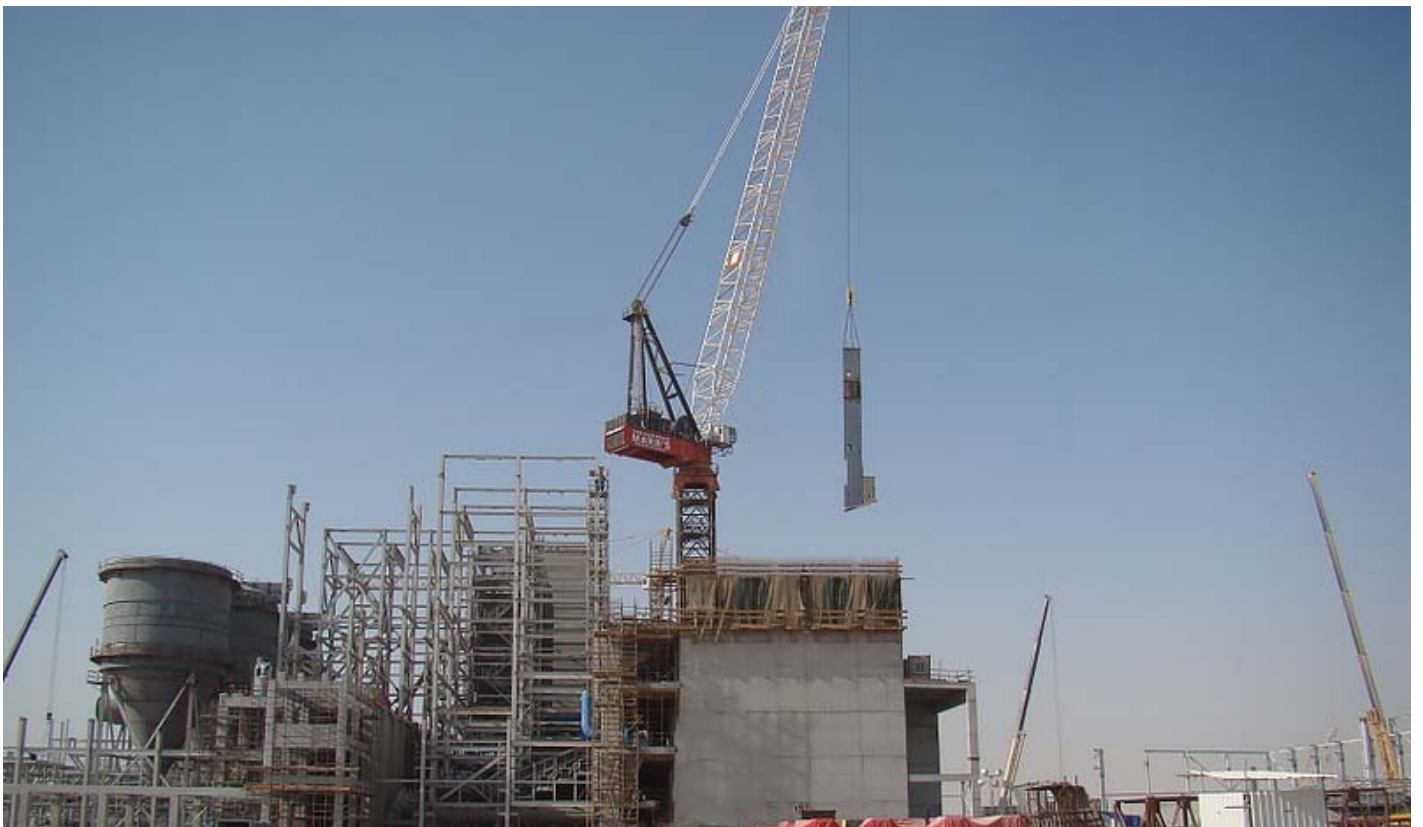
BOILER WALL PANELS INSTALLATION FEASIBILITY DIAGRAM: SHOWING M2480D WITH 74, MAIN BOOM AND 30M FLY, 120 TONNES AT 32M RADIUS.
