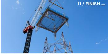
Late August – late October 2021: After completing the lighter lifts at maximum height, Marr's crew climbed the M310D down to its original freestanding height of 117m where it was removed by Marr's Grove GMK6400 and replaced by one of Marr's M1280D Heavy Lift Luffers freestanding on 76m of tower to lift the larger sections and layers of the tower weighing up to 60 tonnes. The project was completed - safely and without incident, three months ahead of schedule.
