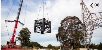
Late June/ early August 2021: Marr's Grove GMK6400 mobile crane installed the M310D tower crane to a freestanding height of 117 meters. Over the next week the crane was climbed to its full height of 193m with an underhook height
