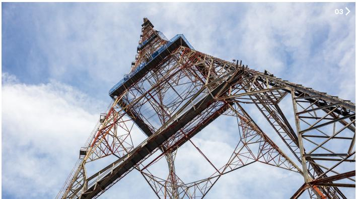
After exploring alternatives including gin poles and helicopters, Mirvac decided on using a crane. However, because the decommissioned tower was not able to accommodate lateral supports, the challenge from a cranage point-of-view was to find a way to get the crane hook height above 233m without the need to build expensive and complicated temporary structures to support the crane.
