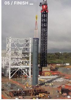
By enabling larger and heavier pre-assembled modules to be assembled at ground level and lifted into position for final connection, Marr's solution created a safer worksite by reducing the risk of working at height.
