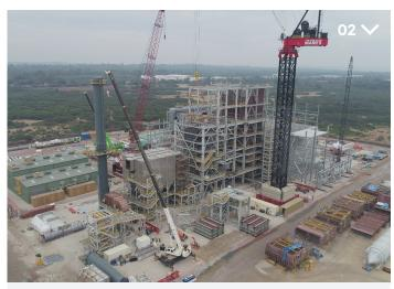
Marr's solution – using a 330-tonne capacity M2480D Heavy Lift Luffer (HLL) stood on one of our ballasted static bases and crane mat system – allowed critical lifts, weighing up to 150 tonnes, to be completed by a single crane from a fixed location.
