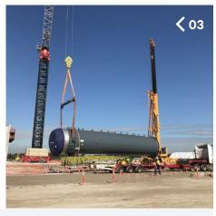
With a total site coverage of over 32,000 square meters and an ability to place 25 tonnes anywhere within the crane's 102-meter radius, we were able to open up areas of the site for pre-assemblies and lay-down which helped to significantly reduce congestion, but still maintained vehicle access through the site.
