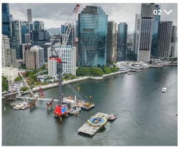
FEBRUARY 2023: With the M2480D installed, the next major lift was installing the 25m x 25m working platform ('megaframe') which weighed over 100 tonnes.
