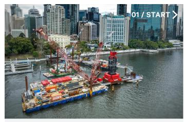
JANUARY/ FEBRUARY 2023: After 12 months in the planning, the first major milestone for us on the project was installing our 330-tonne capacity M2480D heavy lift luffing tower crane on a piled platform in the middle of Brisbane River. The M2480D was installed on one of our ballasted static bases with a barge mounted 400-tonne crawler crane. The M2480D was erected on 16m of tower and then self-climbed to its final construction height of 64m (tower) and approximately 140m of hook height.
