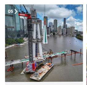
NOVEMBER 2023: After being transported up the Brisbane River by barge, the 180-tonne, 25-metre-tall masthead was installed by the M2480D in a well-planned operation that marked completion of the heaviest and final section of the bridge mast.
