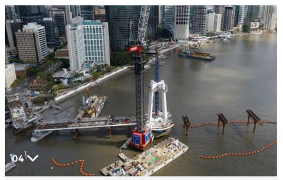
OCTOBER 2023: The unique heavy lifting capacity of the M2480D made easy work of lifting the eight prefabricated sections (four lower and four upper) of the mast legs into place. Each of these prefabricated sections were approximately 25m in length and weighing approximately 40 tonnes.
