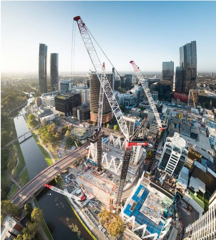
[ABOVE & BELOW LEFT] NSW GOVERNMENT FUNDED PROJECTS - THE NEW SYDNEY FISH MARKETS (MULTIPLEX) AND POWERHOUSE PARRAMATTA (LENDLEASE) WERE THE FIRST CONSTRUCTION PROJECTS IN AUSTRALIA TO USE 100% RENEWABLE DIESEL (HVO100) IN MARR'S CRANES OPERATING ON THE PROJECTS.
